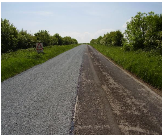
Image Two – New surface & Old surface
