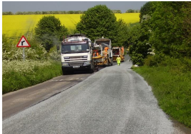
Image One – Chippings being applied
